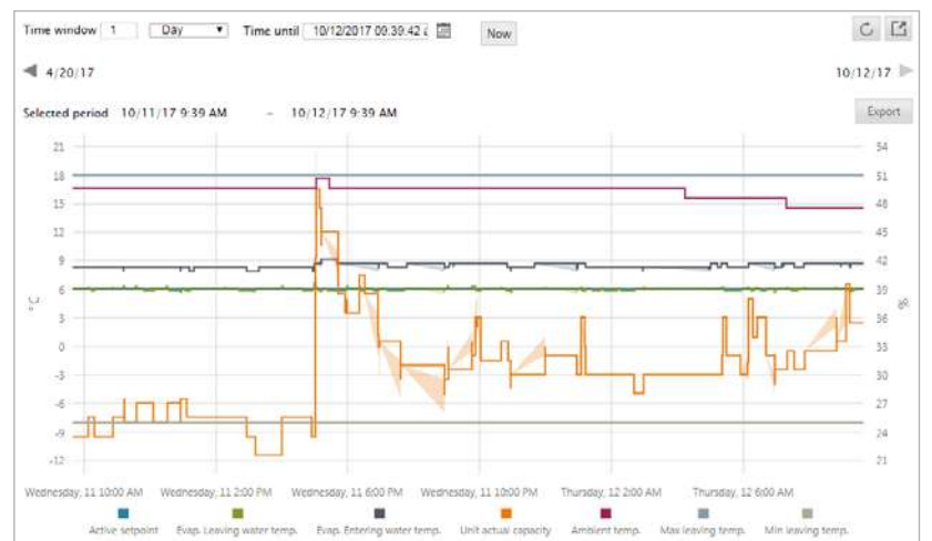
Historical data: select parameters, select period, zoom, ... Full insight in the equipment operation for diagnostics and optimization.
